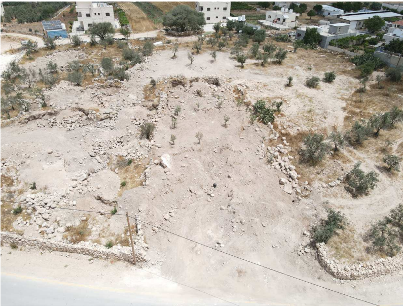
Figure 4. Aerial photograph showing bulldozing of the southern part of parcel no. 1 of Khirbet Qusāṭīn, looking north (photo by Mohammad Abu Nuh).
